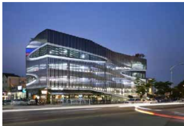
Рис. 2.1. Herma Parking Building
