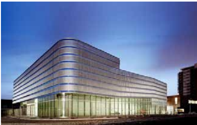
Рис. 3.1. Veranda car park
